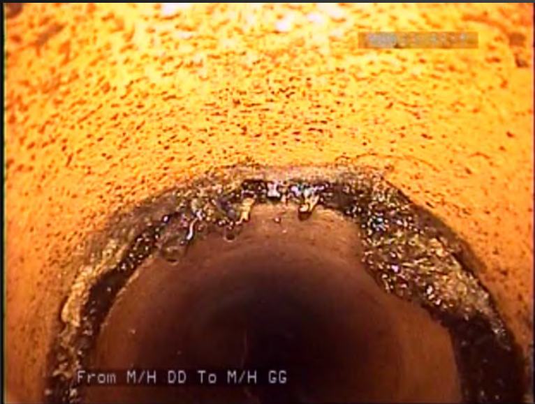
Leaking Joint
