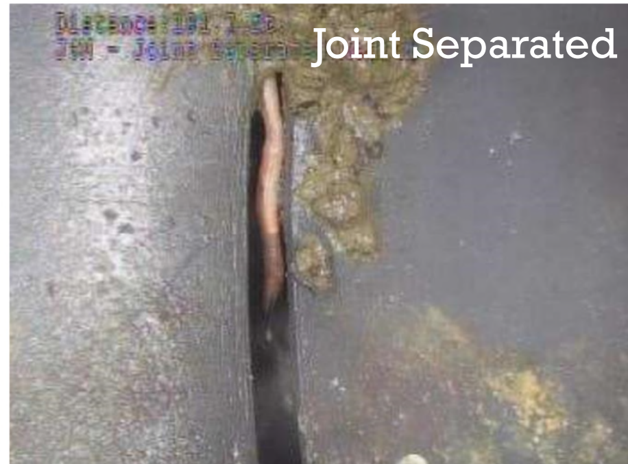
Broken Soil Visible
