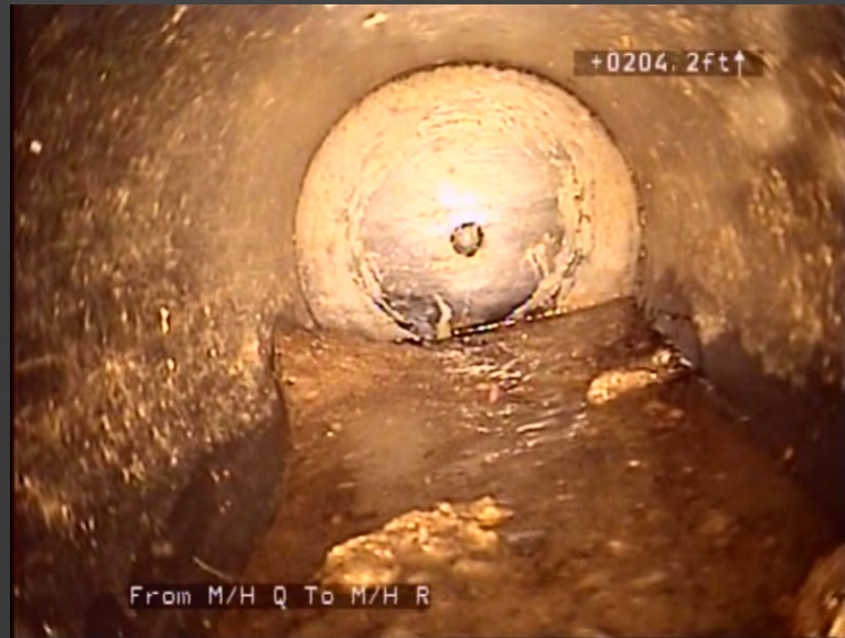
Leaking Stub
