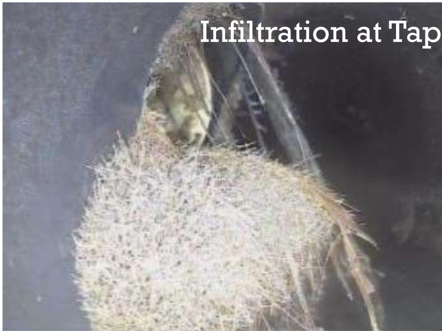
Broken Soil Visible
